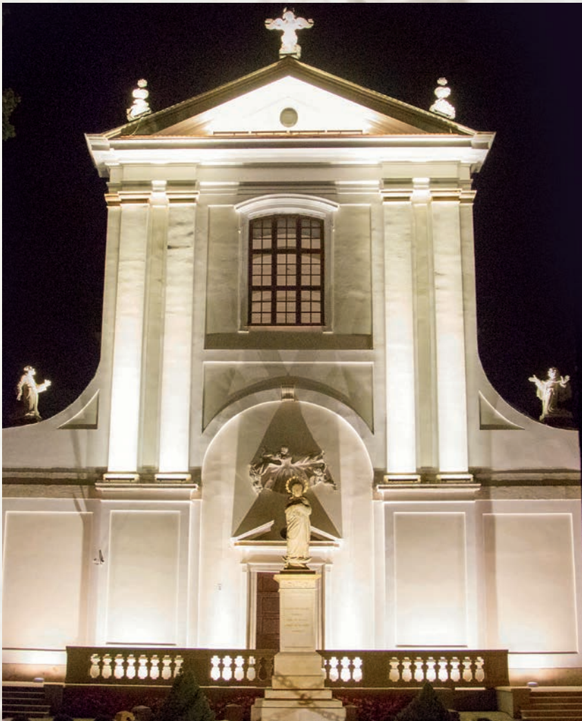
Facade of the post-monastery church in Węgrów. The figure of Christ Seraph is visible in the coping. Photo by P. Buta
