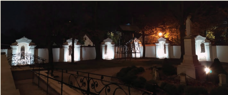
Fence Wall after the renovation-restoration works had been completed. The view at night with illuminated Stations of the Cross (October, 2019). Photo by M. Sobisz
