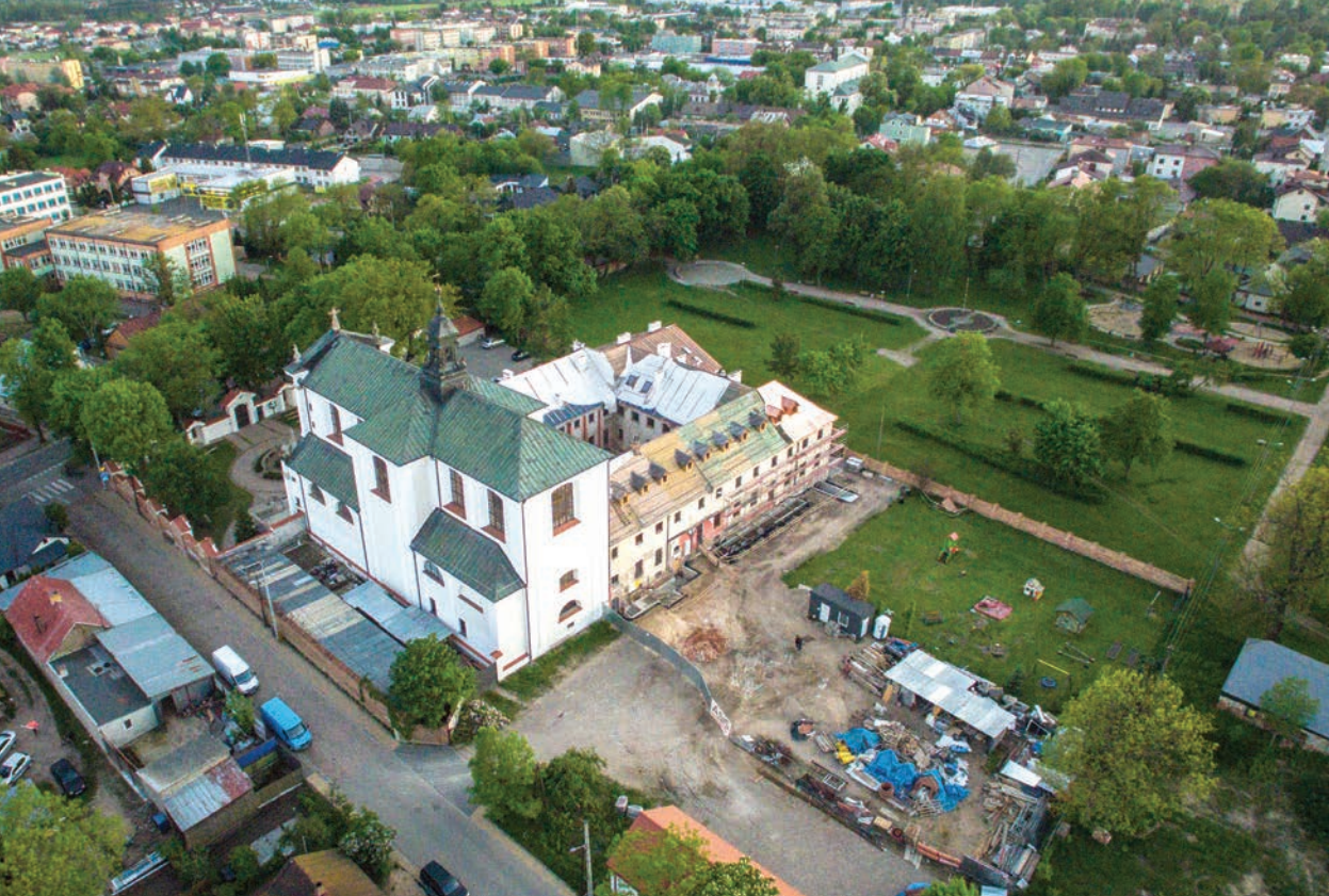
The monastery in Węgrów seen from birdseye perspective. Picture taken when revitalization works had been carried out (June, 2020). Photo by T. Sobisz
